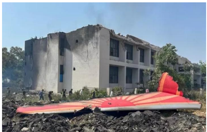
Figure 5 Vertical Stabilizer adjacent to Building A
