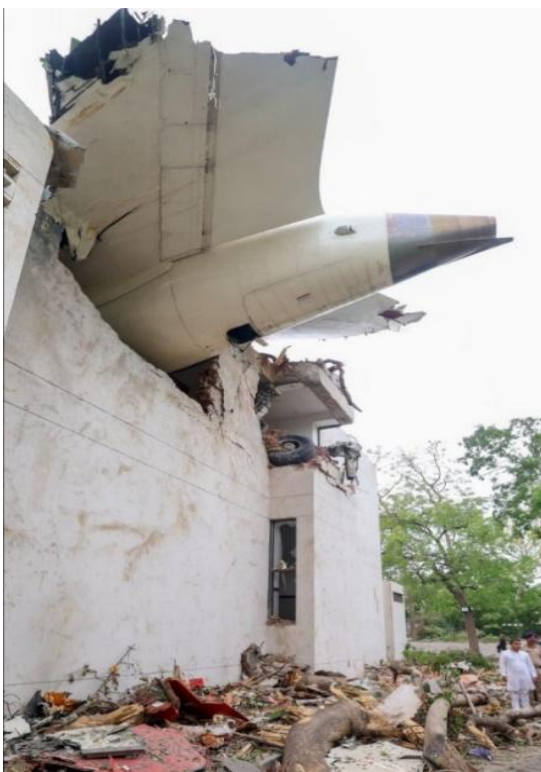
Figure 4 Tail section & RH MLG embedded in the building A
